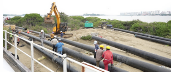
Fabrication and Welding of pipe into sections.
