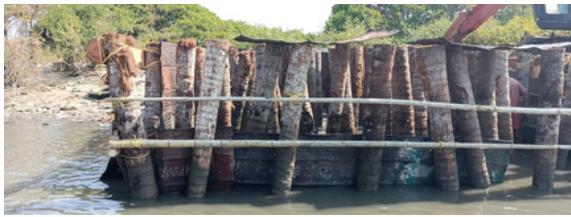
Temporary Jetty Construction using coconut piles.
