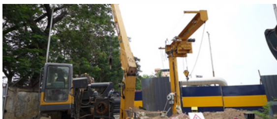
HDD Rigging machine placed on developed area in NJRP.
