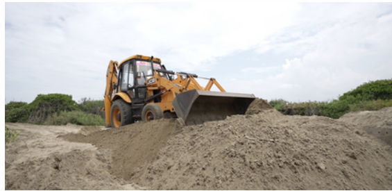
Development of Sandbank Island using dredged sand.
