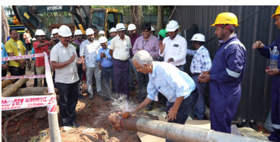
Pooja before commencement of HDD Pilot Drilling
