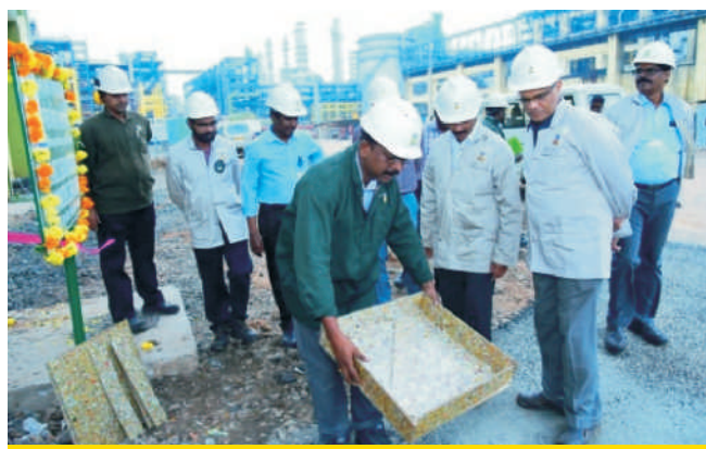
Demonstrating the plastic waste module that is laid beneath the tar
