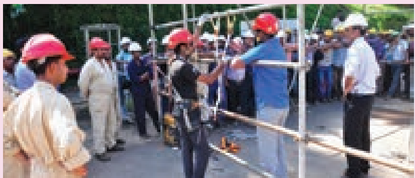
Demo on working at heights in progress
