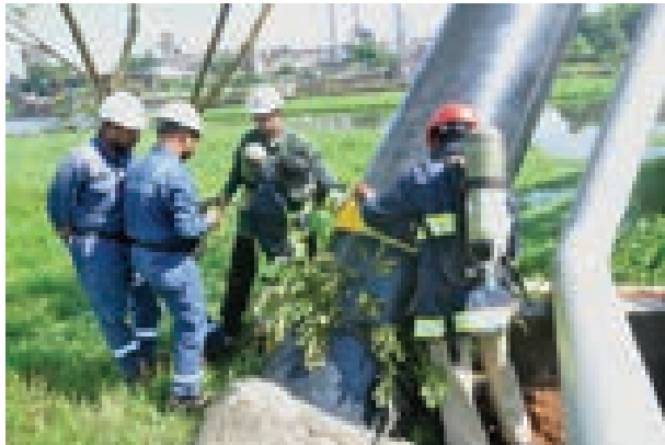
On-site mock drill along cross country pipeline near Chitrapuzha in progress
