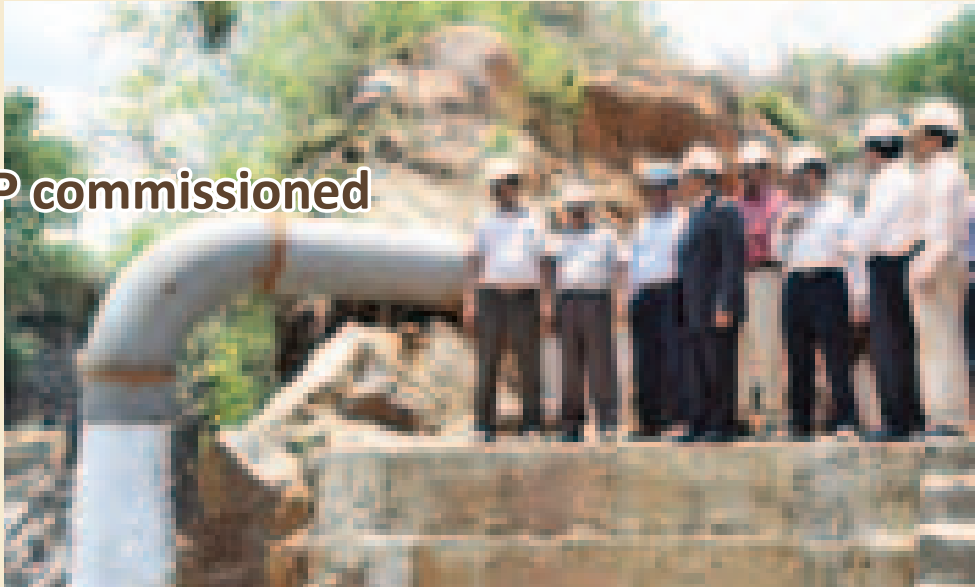
Mr BK Datta, D(R) and senior executives viewing the water inflow from Periyar after inaugurating the facility
